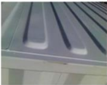
Roof and South Wall Images:
