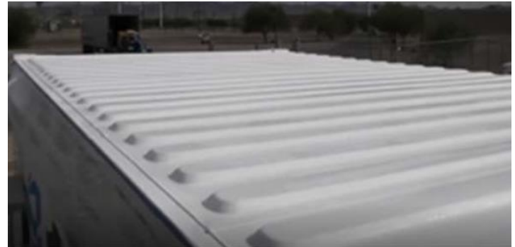
The painted roof of a 20 foot container was dry to the touch within a few hours.
